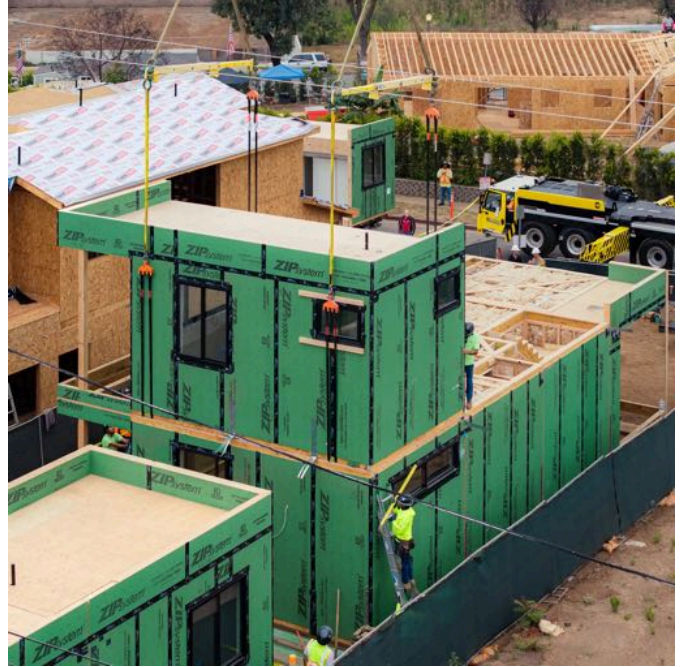
Their new modular home by Marmol Radziner architects being installed
